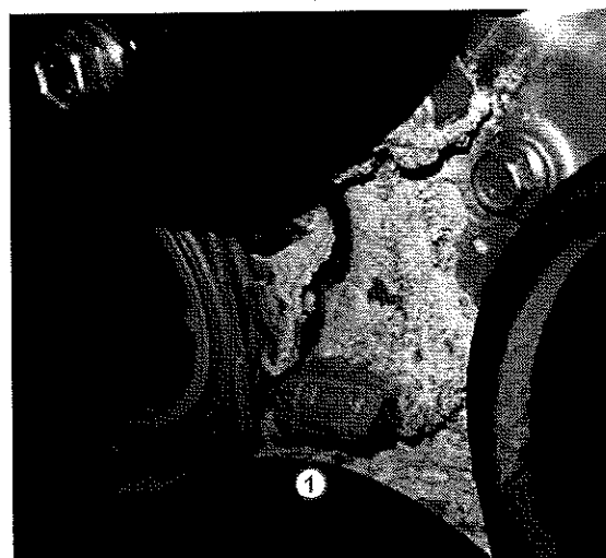
Figure 5. Current Leak – Replace Water Pump
